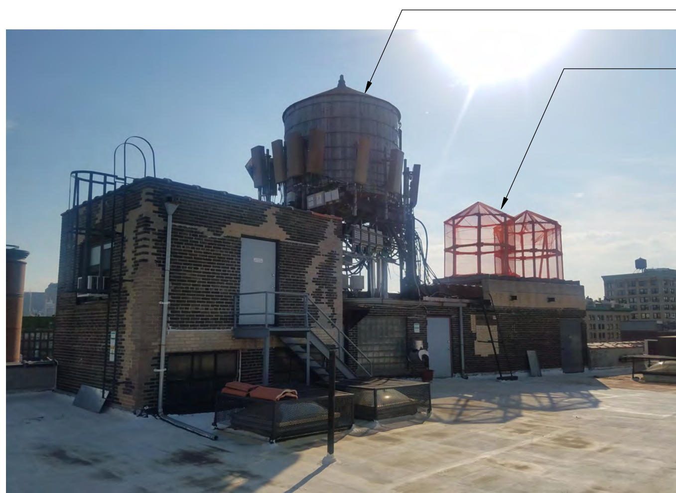
1 EXISTING DOMESTIC WATER TANK WITH (2) PROPOSED SPRINKLER HOLDING TANKS
