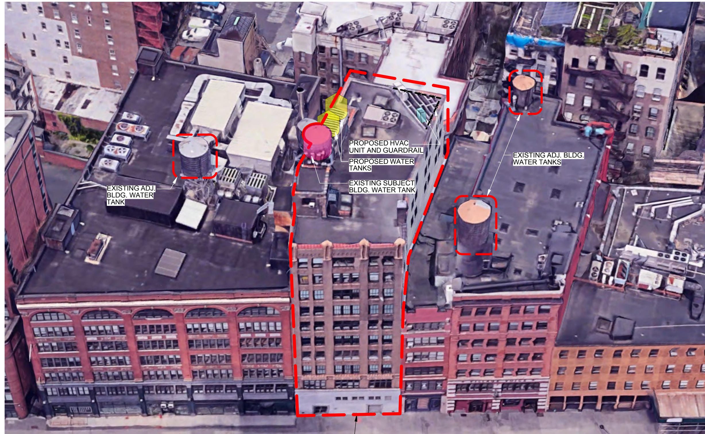
SUBJECT BUILDING 30 COOPER SQUARE
