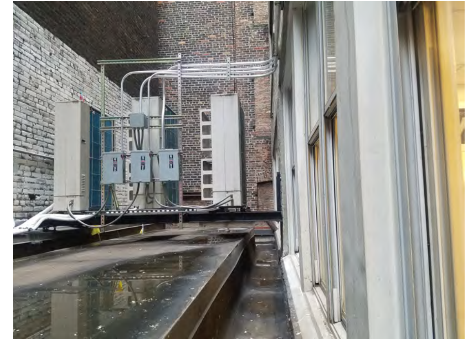
3 PHOTOGRAPH OF 2ND FLOOR ROOF DECK TAKEN FROM 2ND FLOOR WINDOW SHOWING EXISTING HVAC UNITS
