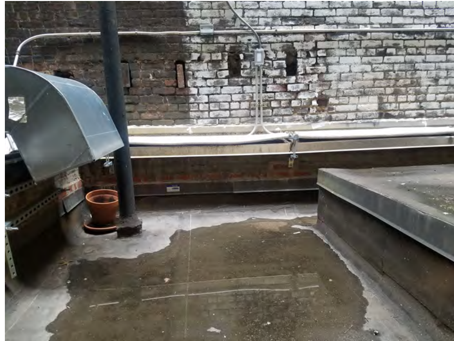
2 PHOTOGRAPH OF 2ND FLOOR ROOF DECK TAKEN FROM 2ND FLOOR WINDOW
